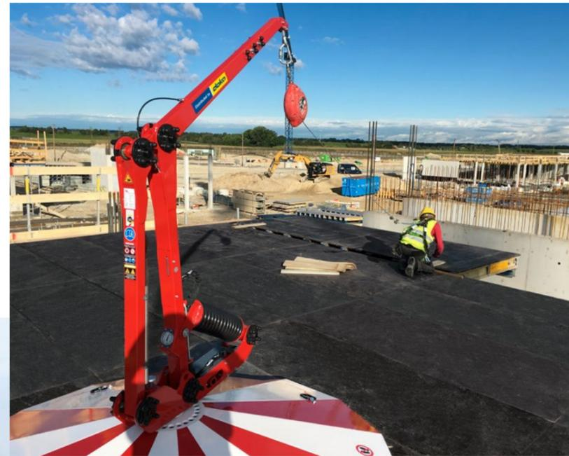
The FreeFalcon protects construction crew members whenever work at drop-off edges is temporarily unavoidable.
