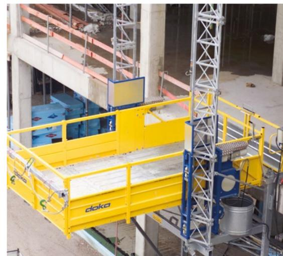
Using the Table Lifting System TLS to reposition tableforms frees up the cranes for other tasks. So it might well be possible to remove them at an early stage and proceed with work on the outdoor facilities.
