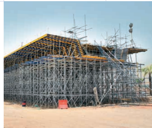
▲ High-capacity and high-performance Staxo 100 for shoring and structural support.
