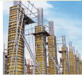
▲ Universal Frami Xlife panels are ideal for varied cross-sections of column in a 5 cm grid – including forming special 6 m columns.
