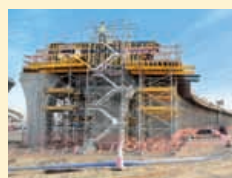
JLT Bridges Dubai
