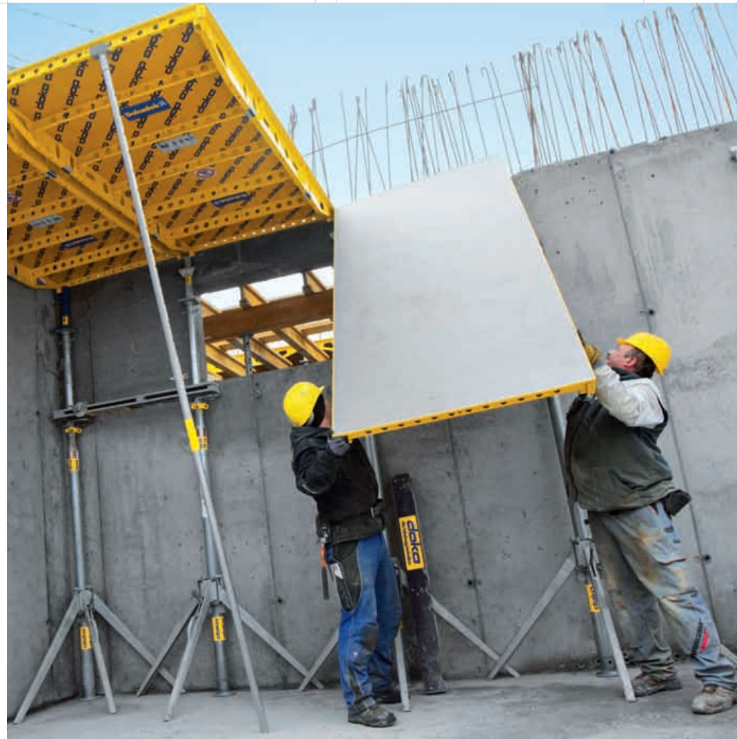
▶▲ Virtually error-free erection as the Dokadek 30 system has only three different components: panels, heads and props.
