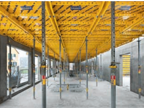
▶▲ Virtually error-free erection as the Dokadek 30 system has only three different components: panels, heads and props.
