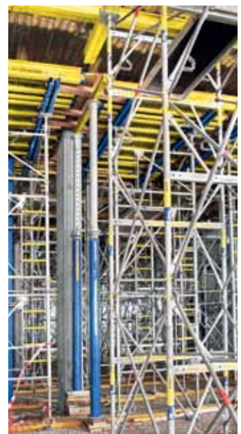
▲ Doka's Eurex 60 prop, in combination with Staxo 100 and Staxo 40 for infill solutions, makes forming a lot easier.
