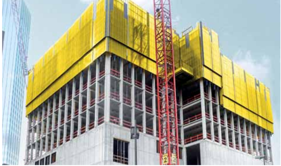
Photos: Tainus Turm, TismannSpeyer, Frankfurt/Main, Germany Contractors: Ed. Züblin
