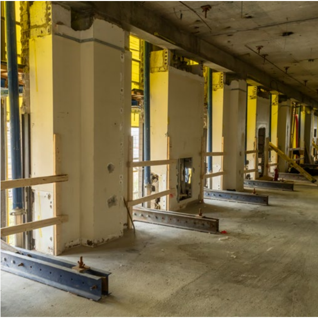
Flexible Height Adjustment to Individual Demolished Areas: The protection screens can be lowered progressively as each floor is cleared, maintaining safety throughout the demolition sequence.
