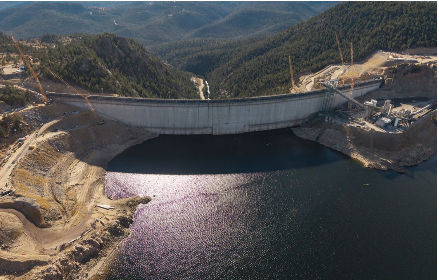
The Gross Reservoir expansion is on track for completion in 2027.
