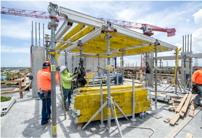
Four and Done: With only four main components—joists, stringers, drop head, and props—SuperDek reduces inventory complexity on the community-focused build.
