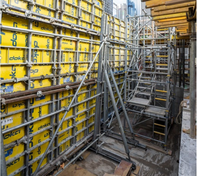
Interior platforms carry stair towers for safe deck access.
