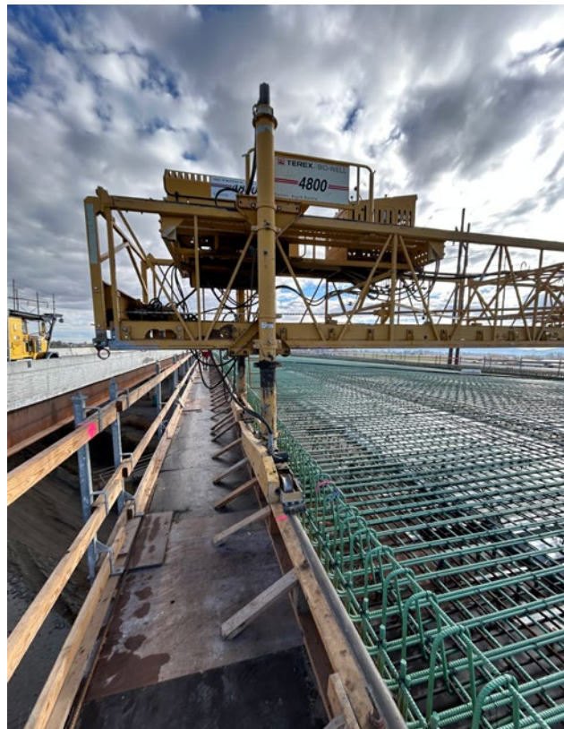
Hanger Hangup: In less than a month, Doka custom-designed hangers to support the bridge rework.
