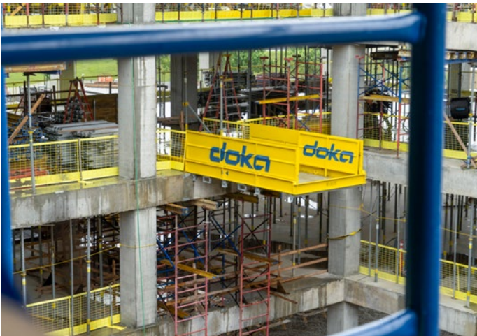
Logistics Partner: Doka Loading Platforms serve as temporary work decks where materials and equipment can be staged safely.
