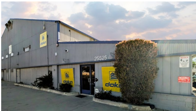
New Doka facility in Loma Linda, California.
