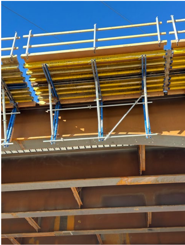
Modular Mix: ParaTop's modular design proved ideal for the I-84 Heyburn interchange, adapting to the bridge's varying geometries while creating clean, accessible workspaces.
