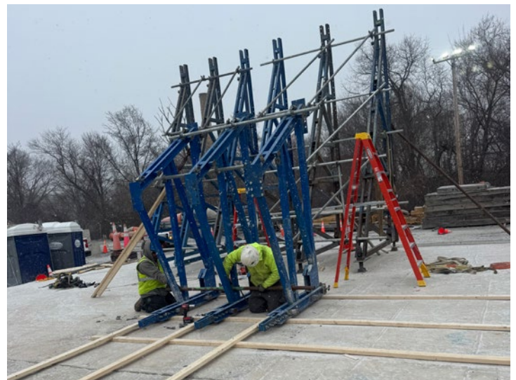
Aligned, Accessible Efficiency: Doka D22 supporting frames ensuring proper alignment and load distribution.
