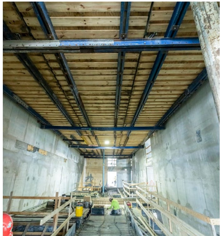
Strength & Accessibility: The Super Climber formwork solution includes double gantry beams bolted together across the core provides the structural foundation for the belt wall, while keeping lower levels accessible.
