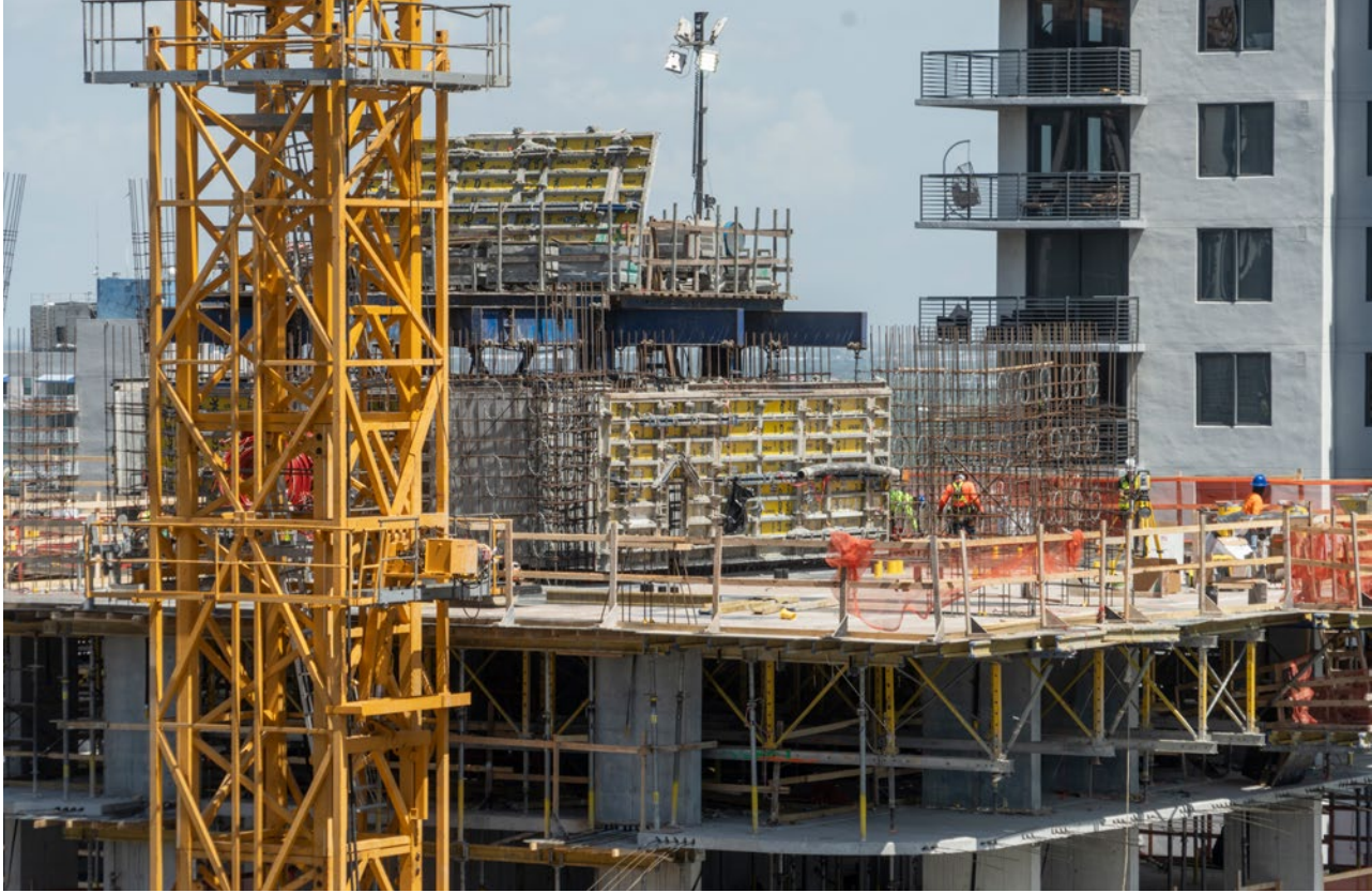
Advanced engineering execution showcasing the SuperClimber system Framax wall formwork and Truss tables working together to optimize construction performance.
