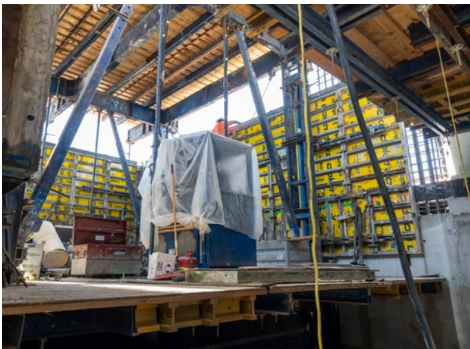
Strength & Accessibility: The Super Climber formwork solution includes double gantry beams bolted together across the core provides the structural foundation for the belt wall, while keeping lower levels accessible.
