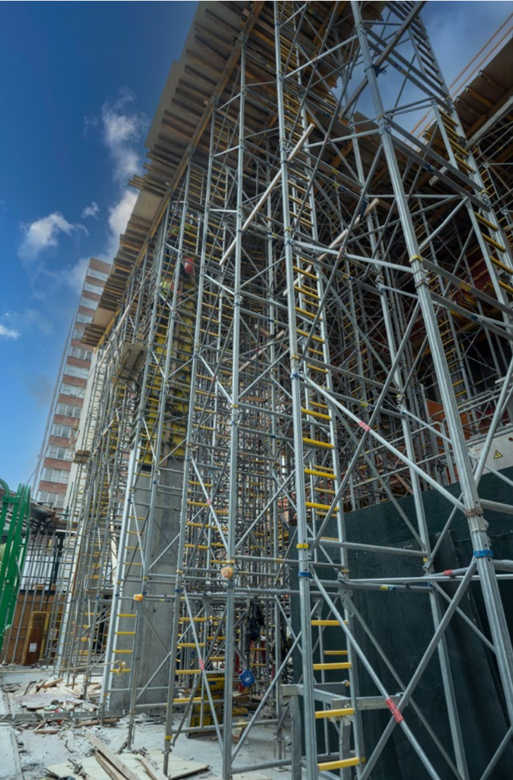
Slab Support: Staxo 100 shoring systems supported slab forming of substantial concrete beams and extreme heights in various areas of the project.
