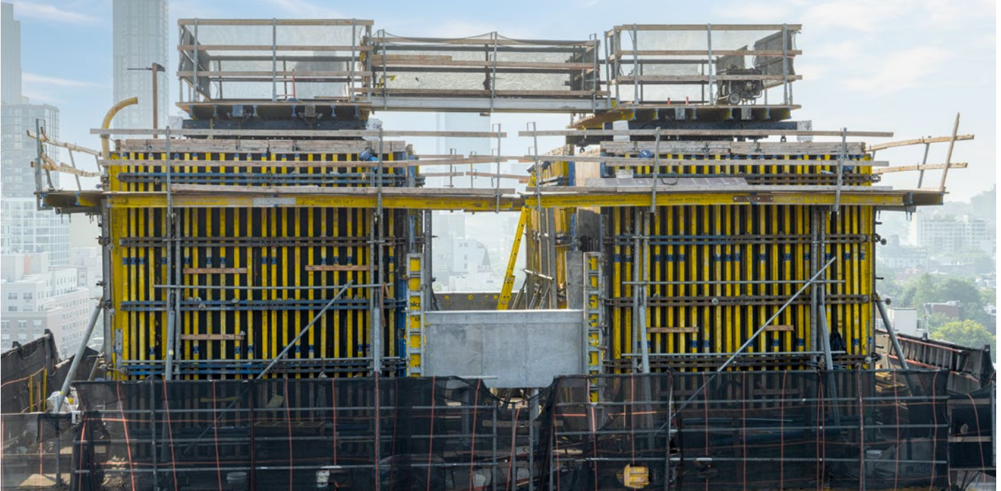
Dual Core Advancement: Both towers rise simultaneously, their different climbing approaches working in parallel.
