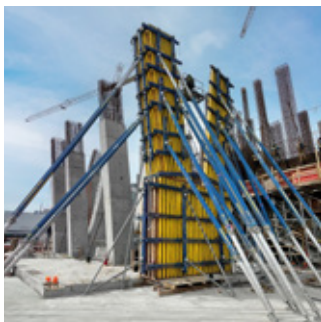
Tall walls and columns
