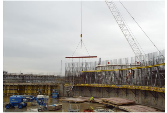
Prefabricated Reinforcing cage being lifted into position
