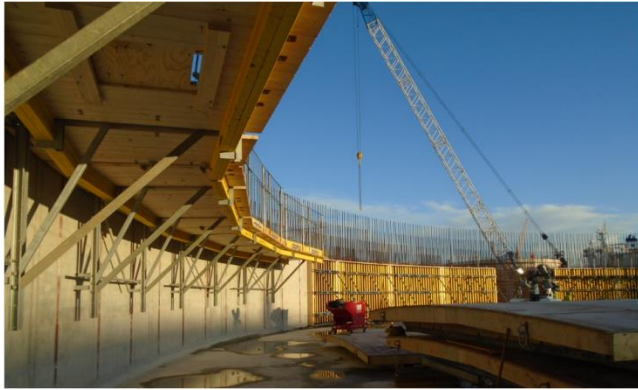
Doka MF240 Platforms fixed in place ready for 2 nd lift pour
