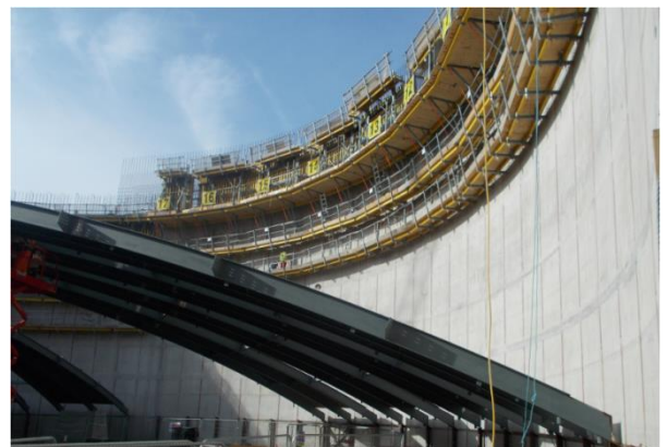
Internal Doka MF240 Climbing platforms & Top 50 Circular Formwork
