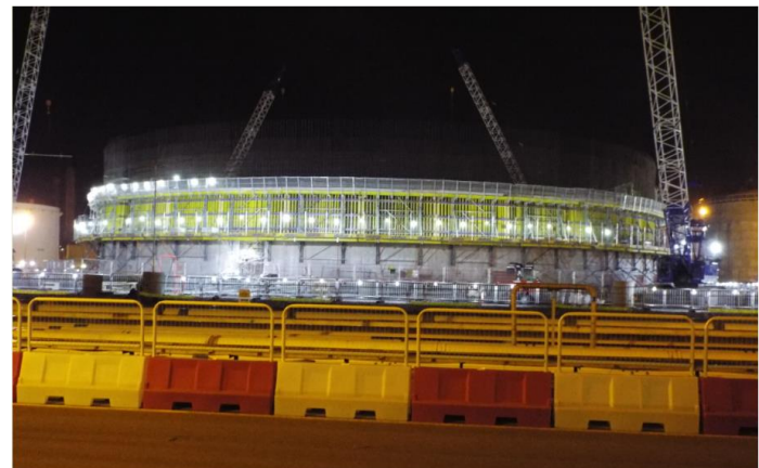
67.5 m diameter Ethane tank under construction
