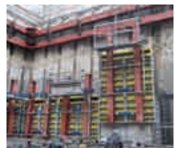
▲ An earth retaining unit is 2.4 m in width and 2.7 m in height.
