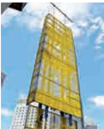
▲ Protection screen Xclimb 60 with Framed enclosure Xbright was pre-assembled and used at a project in Sydney CBD.
