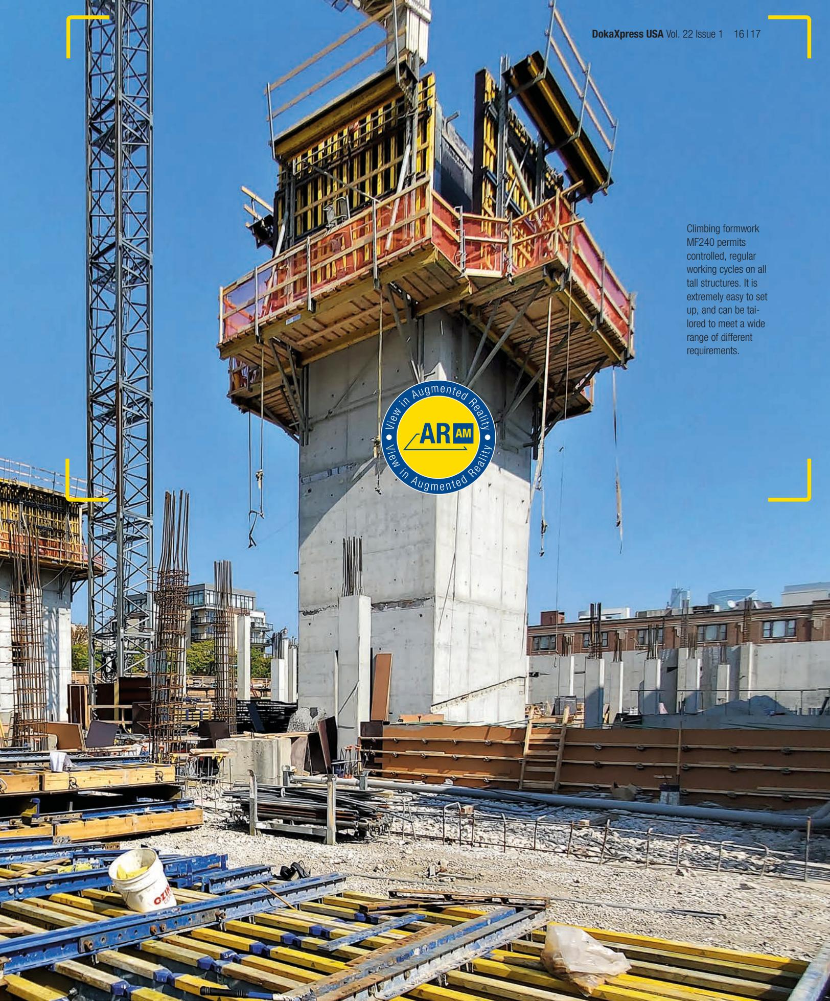
Climbing formwork MF240 permits controlled, regular working cycles on all tall structures. It is extremely easy to set up, and can be tailored to meet a wide range of different requirements.
