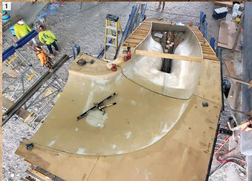
The concrete staircase is designed so that it appears to float up to an intermediate landing and curve into a turn to continue upward to the second floor. Doka engineered the custom stair formwork for Nashville-based contractor Charter Construction. The specially designed formwork made the construction of the architecturally demanding staircase relatively effortless.
