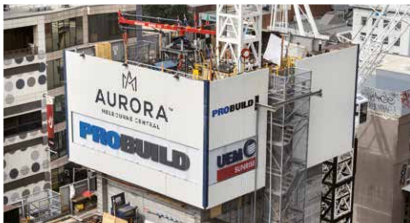
▲ The lead Lubeca System for the Aurora Project, including allowance for crane and palcing boom.
