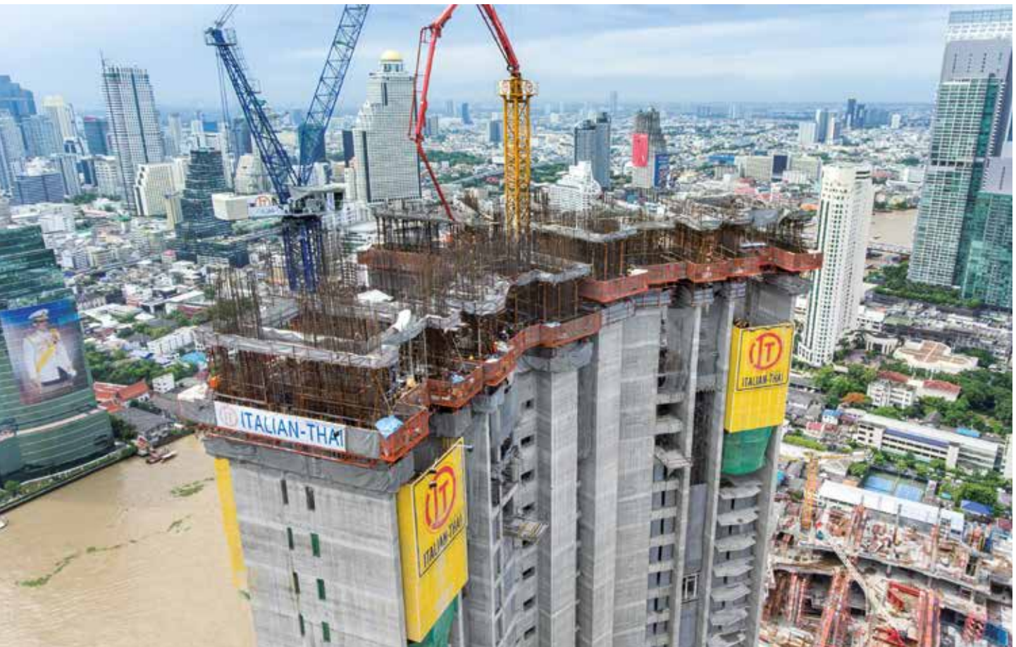
▲ Customer branded Protection Screen Xclimb 60 for safe working conditions at Icon Siam Tower “The Magnolias Waterfront Residences”.
