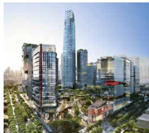
▲ Topping out at 492 metres, the Exchange 106 will be another architectural highlight in the skyline of Kuala Lumpur.
