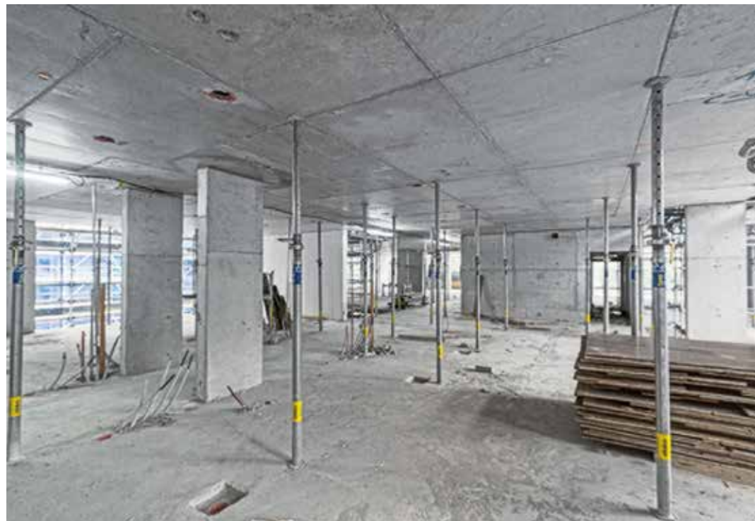
▲ Uniform and clean concrete finish after stripping the formwork.
