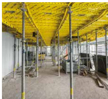
▼ Reduced use of props thanks to Dokadek 30.
