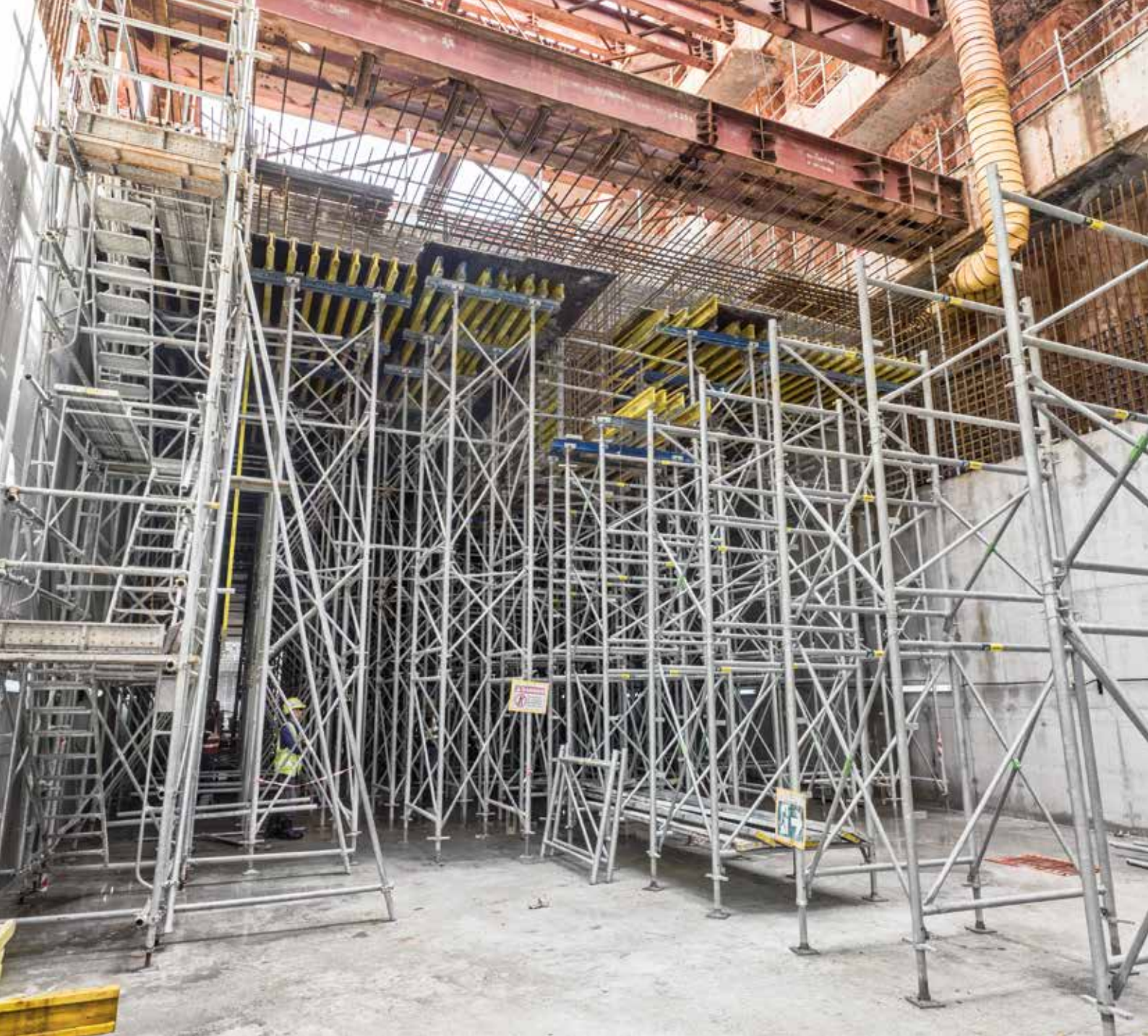
▲ Doka d3 load bearing tower system used for slab construction.
