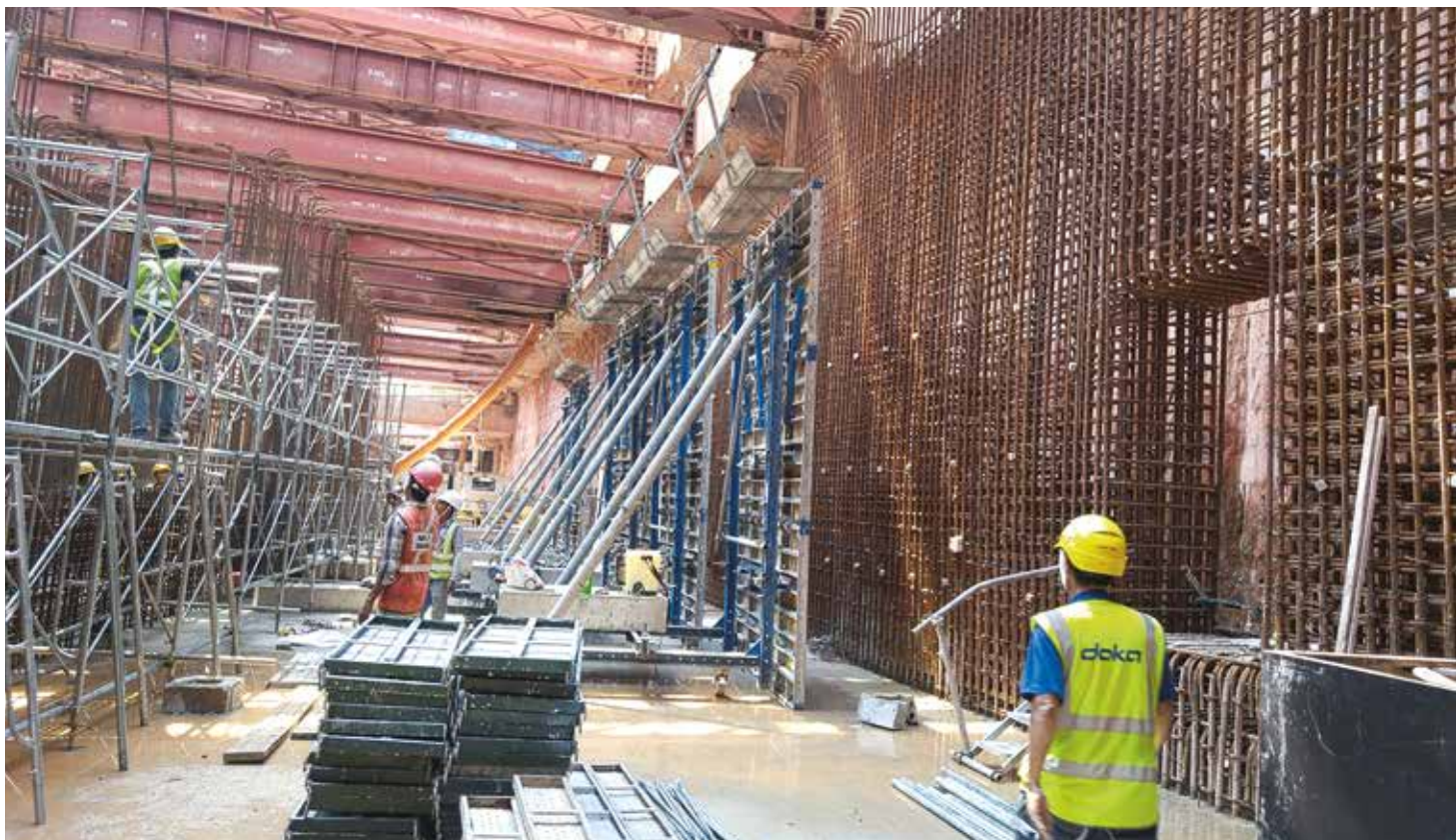
▼ Doka d3 load bearing tower system used for slab construction.
