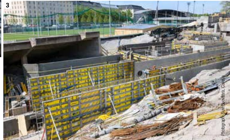
In order to support all these structures, a total of 13,000 Staxo 100 frames and over 10,000 arch supports were used. Additionally, an enormous range of different machinery was used. In the main, the Framax Xlife wall formworks are utilised, but special surfaces have also required use of the Top 50 formworks that were assembled at the construction site.
