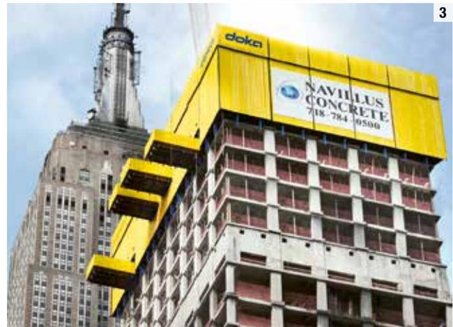
sure particularly safe working. The excavation safety device integrated into the Dokadek 30 head prevents elements from falling down accidentally.
