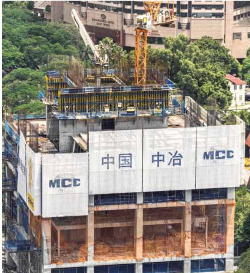
▼ Safe working conditions are assured by the Protection screen Xclimb 60 with a perforated trapezoidal sheet.
