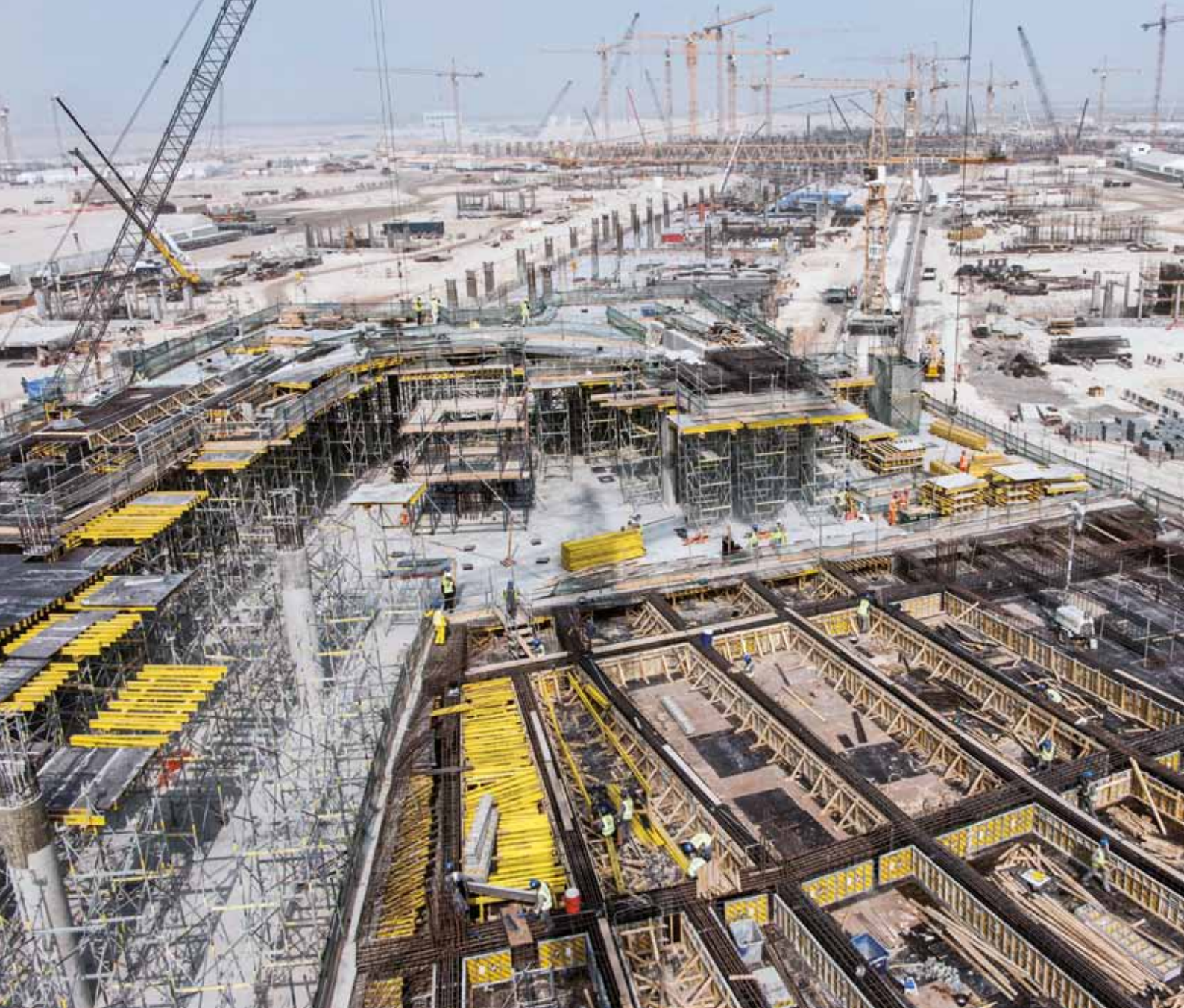
▲ Doka Abu Dhabi developed a customized formwork solution for the expansion of the international airport in Abu Dhabi.
