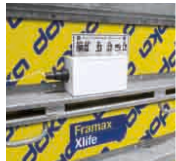
▲ Wall sensor and slab sensor during application
