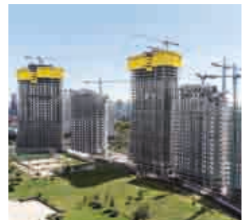
▲ Doka developed the formwork solution for the five highest skyscrapers.
