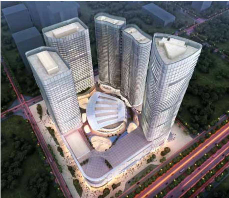
▲ The center will consist of five super-highrise towers and high-end business premises. Doka supplies formwork for the highest building.
