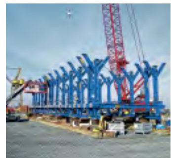
▲ Preparations for the immersed Second Midtown Tunnel are underway in the dry dock.
