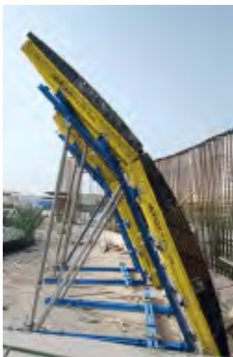
▲ More than 1,800 m 2 of Large-area formwork Top 50 are in use at the Kahramaa Awareness Park.
