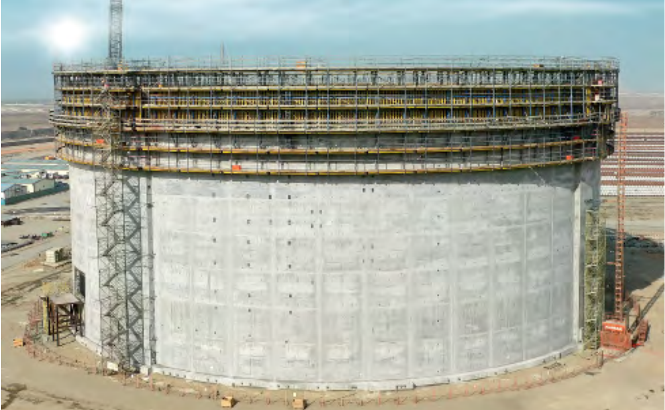
▲ For storage structures such as LNG tanks or silos Doka offers preferred solutions of self-climbing or crane-lifted climbing formwork systems with safety as the top priority.
