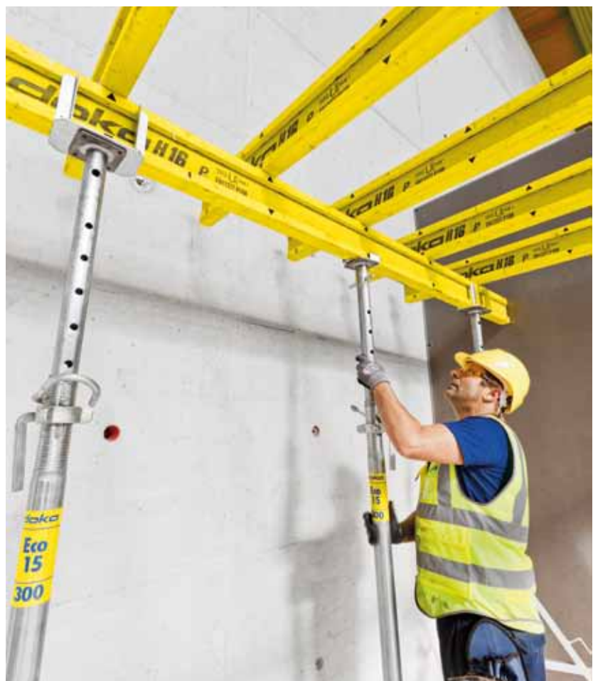
▼ Dokaflex 15 has been developed specifically for forming concrete floor-slabs of between 10 and 15 cm in thickness. This versatile hand-set system features weight- and capacity-optimised system components and so is very easy to handle.
