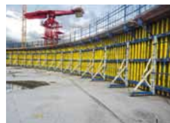
▲ First step of inside formwork are support by Scissor-action spindle and special starter. Inside the job site is clean and tidy.
