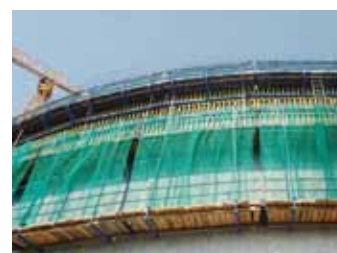
▲ All suspension platforms are protected by safety net.
