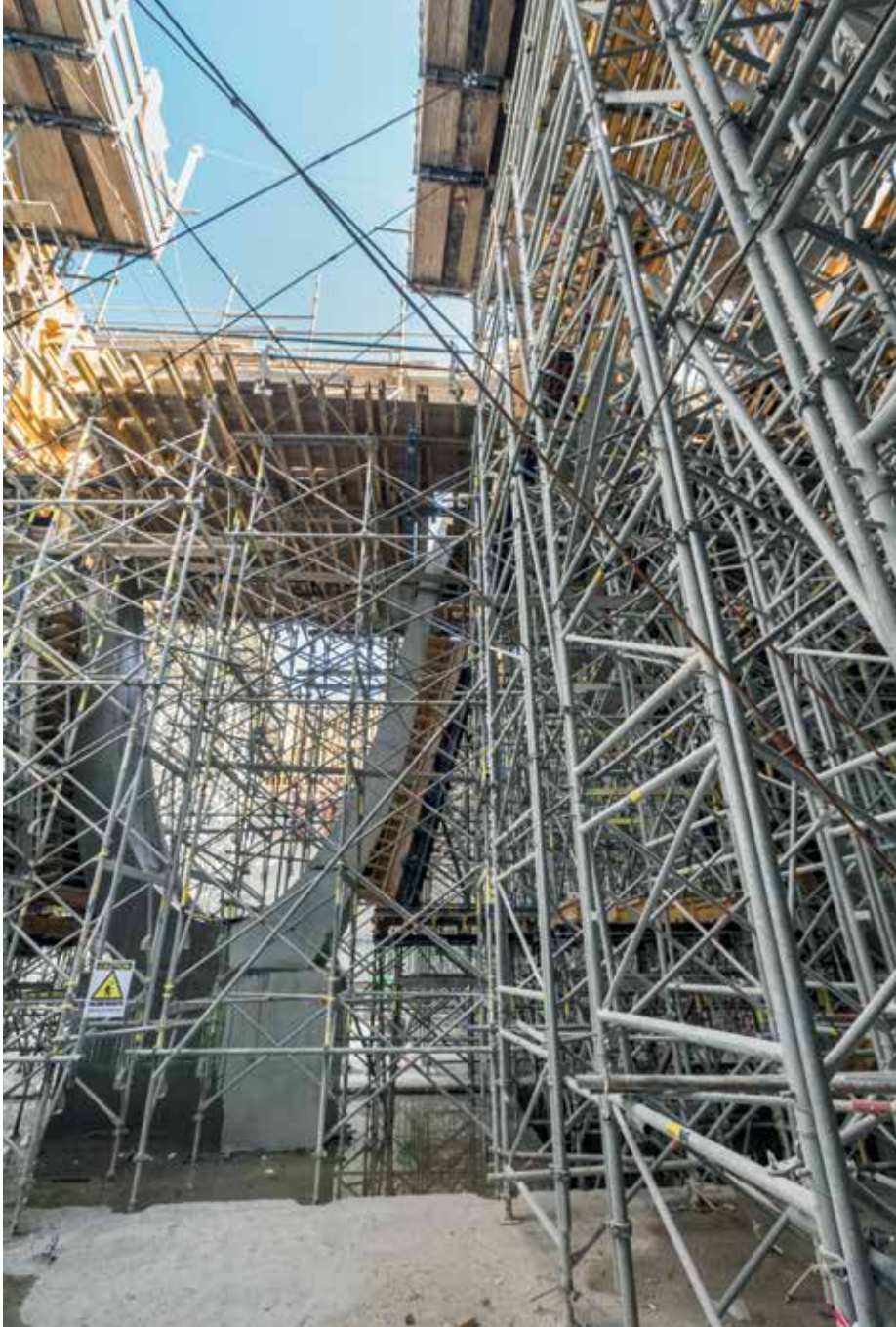
▲ Doka Qatar assembled and designed 6,000 m 2 of formwork for this project.
