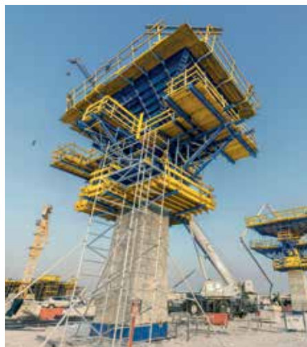
▲ The robust structure of pier head steel moulds can be reused on multiple occasions and provide a higher quality concrete finish.
