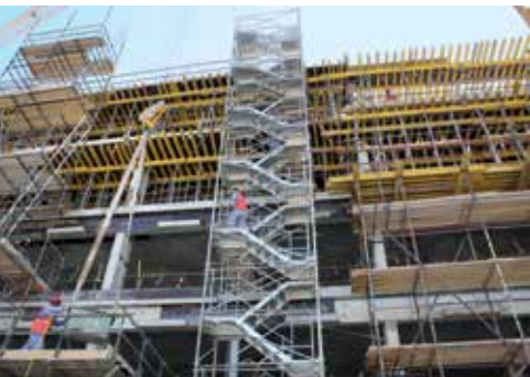
▲ Doka's easy to erect d2 stair tower assures safe and fast building access at each floor, even at heights of over 40 metres.
