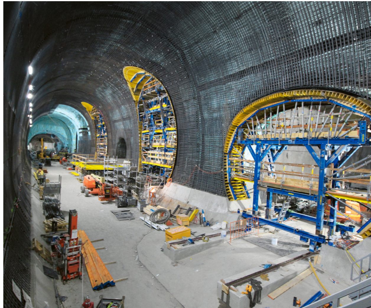
Tunnelling formwork at Sydney Metro Doka's extensive experience in tunnelling and metro construction have made it the preferred choice for mass transportation projects throughout the region.
