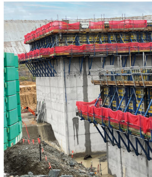
Dam formwork D22 and Framax Xlife in position on Rookwood Weir.
