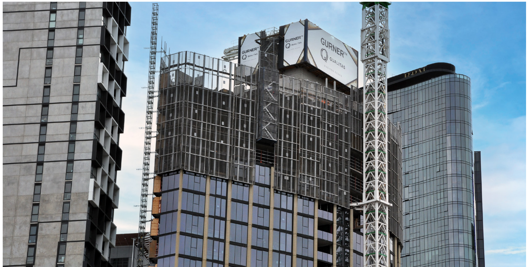
Lubeca Jumpform in action at Madison Grand project in Melbourne.
