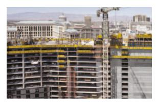
Safe choice, right system: The Automatic climbing formwork SKE is definitely the safe choice of system. Its wide, fully railed-in working platforms, which can be completely enclosed over the entire area if desired, give your site the ultimate in safety.
