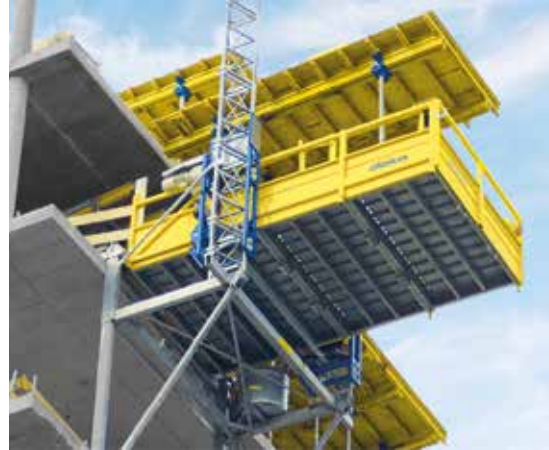
Fast construction workflows without the crane: with the Table Lifting System TLS, tableforms are brought up to the next floor at the push of a button.
