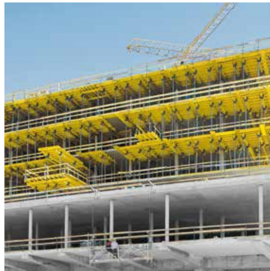
Even with large-area floors, Dokaflex tables ensure rapid construction progress thanks to custom-designed concrete props.
