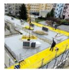
• fast stripping made possible by panels that are easily and safely tilted
