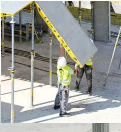
Quickly forming up to 3.50 m room height without aids working safely from floor-level
