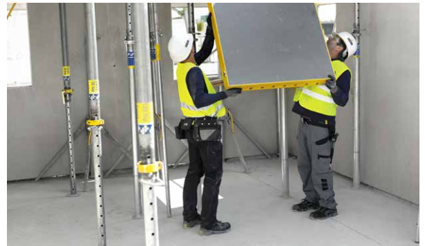
The DokaXdek panel floor formwork is a lightweight and flexible two-person element system.
