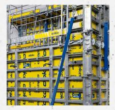
Panel struts on the formwork (with formwork-adapter pin set and panel-strut shoe)
