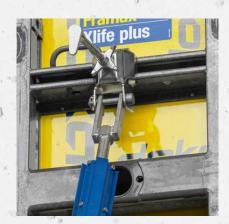
Alignment strut on the formwork (with formwork-adapter pin set)
