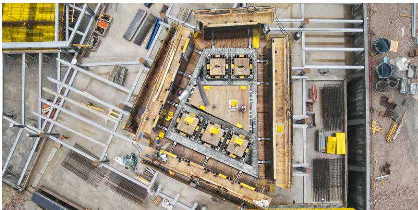
With the shaft system, even small-celled shafts – of any shape – can be formed independently of the crane.
