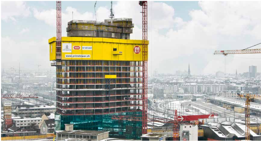
SKE50 plus is the easiest and also the most flexible system in the Doka automatic climbing portfolio.
