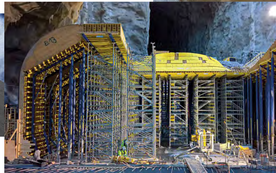
← Vamma Power Station, Norway One of the biggest hydraulic power expansions in Europe since the 1980s needed special formwork from the Doka pre-assembly service for the draft tube. 1,500 m³ water per second will flow through the 12 turbines of the power station.
