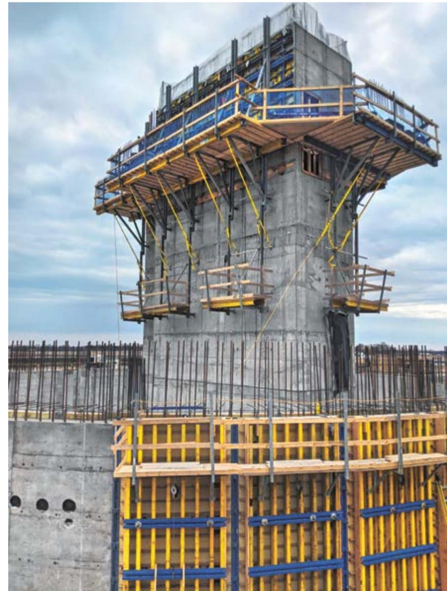
1 Framed formwork Frami Xlife in combination with climbing formwork MF240 on the outside of the building core.
