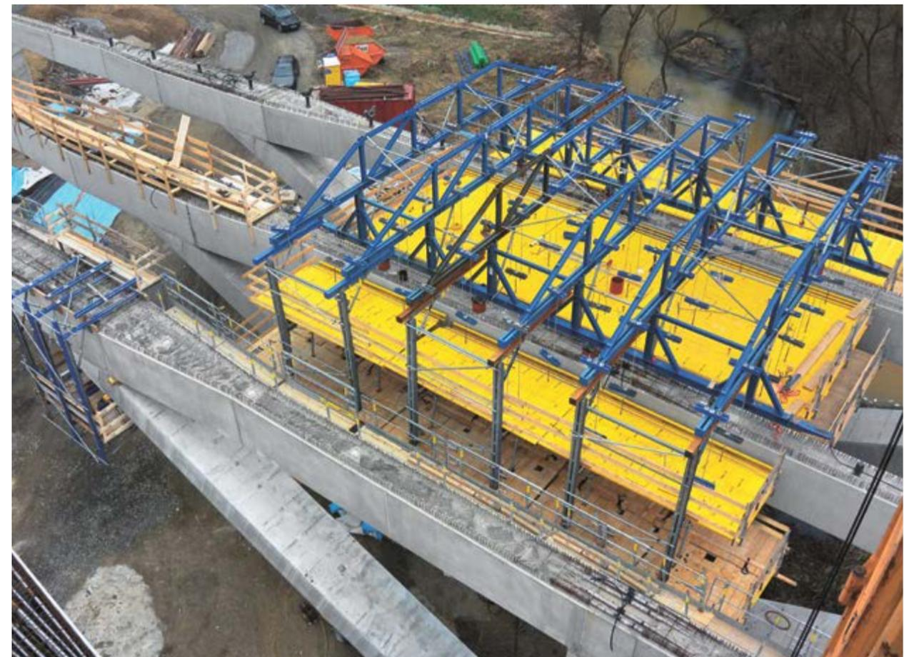
1 The folding bridge method does not require any falsework, which saves time and money.
