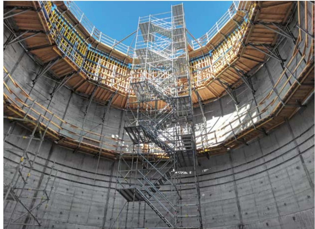
1 The large-area formwork Top 50 elements were made to a custom height so the entire clarifier could be poured in five lifts.
