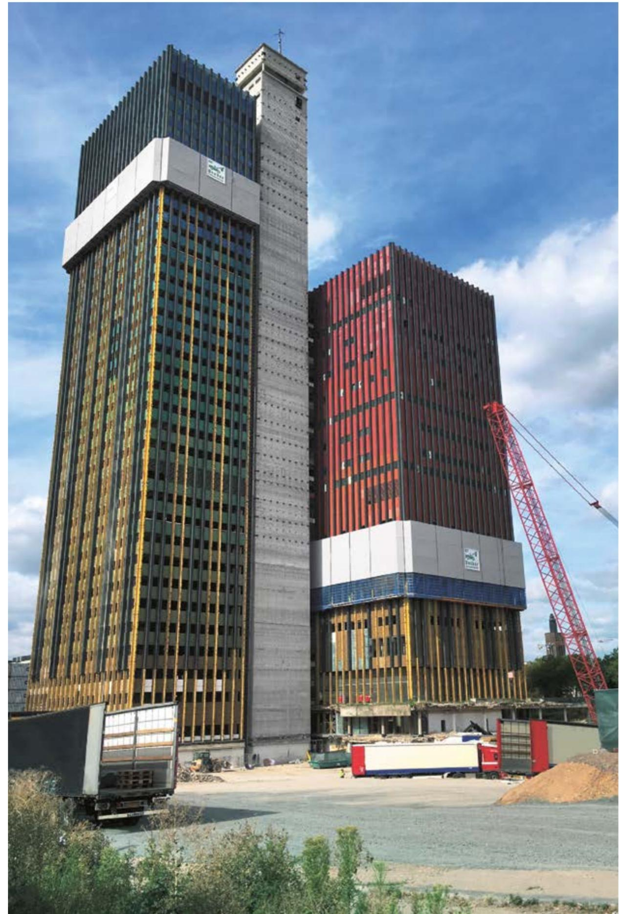
The office tower (left) and the studio tower were fully enclosed with the protection screen Xclimb 60 for dismantling.
