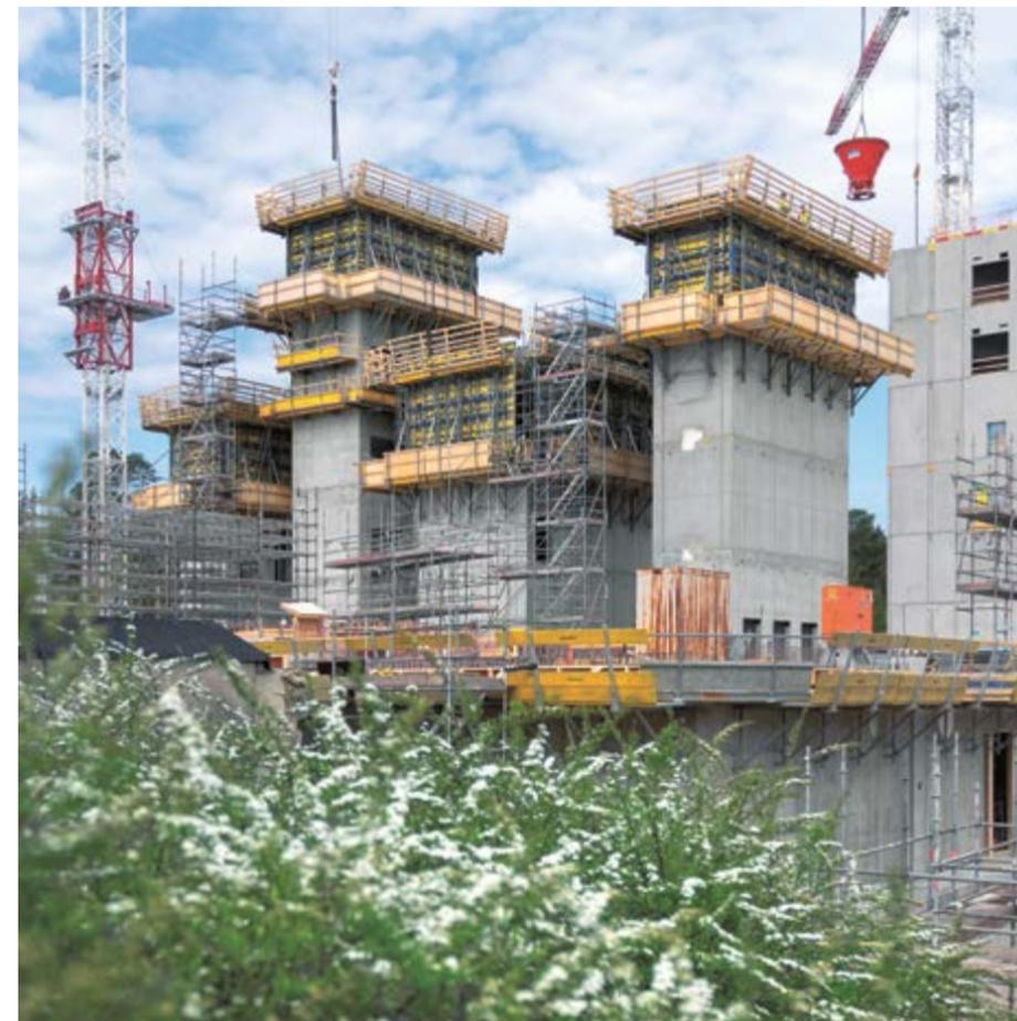
1,2 Building B of the hospital is being realised with the climbing formwork MF240 and the framed formwork Framax Xlife plus.
