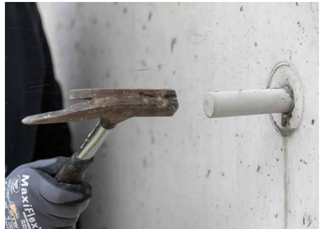
2. Tap the concrete cone into the form-tie hole from the bigger side
