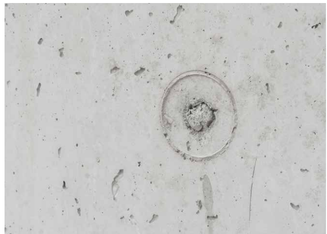
4. Form-tie hole fully closed
