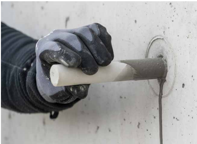
1. Coat the concrete cone with cement slurry or adhesive and insert it into the form-tie hole
