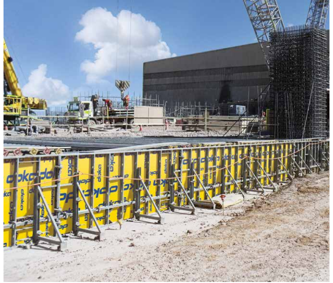
Even extended alignments do not require additional stiffening.
