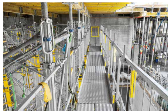
The assembly platform offers an extended access to the superstructure without compromising the system flexibility or performance.
