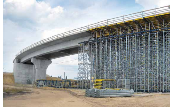
The robust Staxo 100 steel frames demonstrate their high load-bearing capacity in free-standing use.
