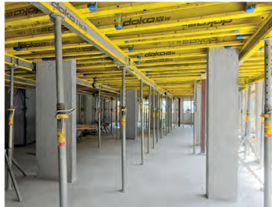
The wide spaces left between the floor props, and the fact that far fewer system components are needed, make for fast workflows.
