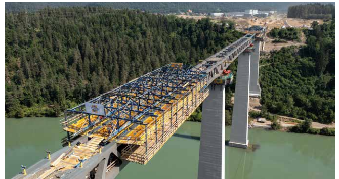
Jauntal Bridge, Austria. High work safety at a height of 96 m and individual adaptation of the formwork to the steel structure ensure smooth construction progress.
