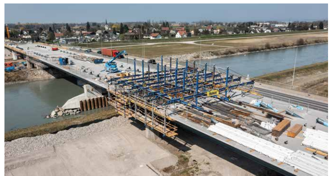
Rhine Bridge Hard-Fussach, Austria. Customized composite formwork carriage with two longitudinal trusses and two additional rows of pendulum props enables the construction of this exceptionally wide and asymmetrical cross-section.
