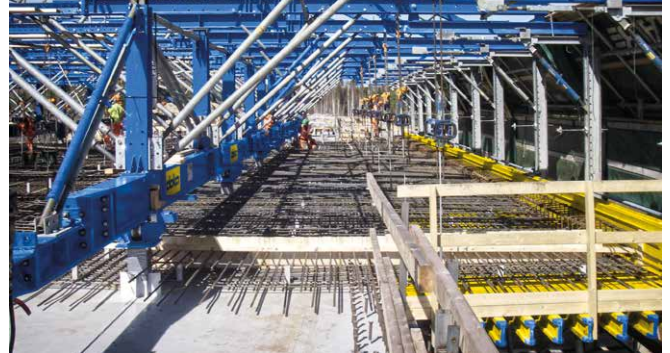
The System beam NG allows the Composite forming carriage to be adapted to the structure geometry even more flexibly.
