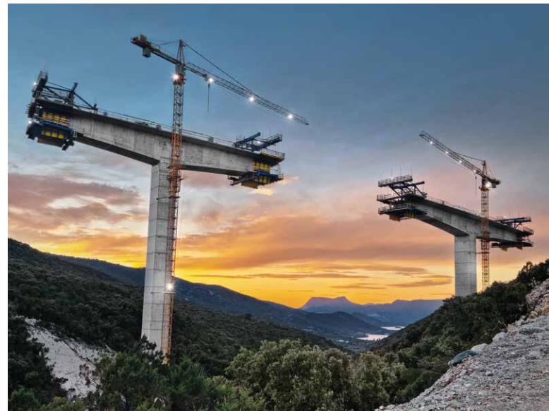
Dumanja Jaruga bridge, Croatia
