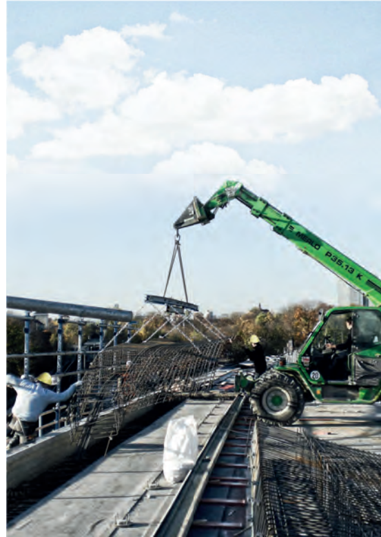
Pre-assembled reinforcing cages can simply be hoisted into place from above.
