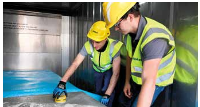
Concremote as part of the prototype development of the Intelligent Heated Formwork
