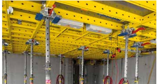
Test construction site in Trondheim, Norway
