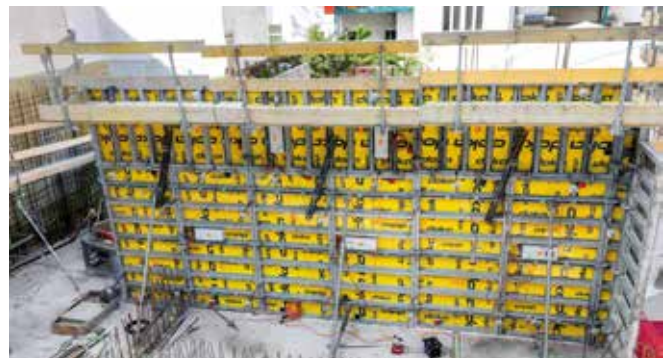
Test construction site in Vienna, Austria
