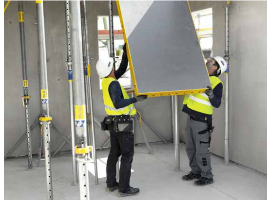
The DokaXdek panel floor formwork can be safely assembled from the ground.
