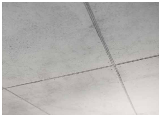
Good concrete result
