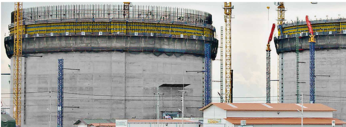
Climbing formwork 150F in use with two large LNG tanks in Thailand.
