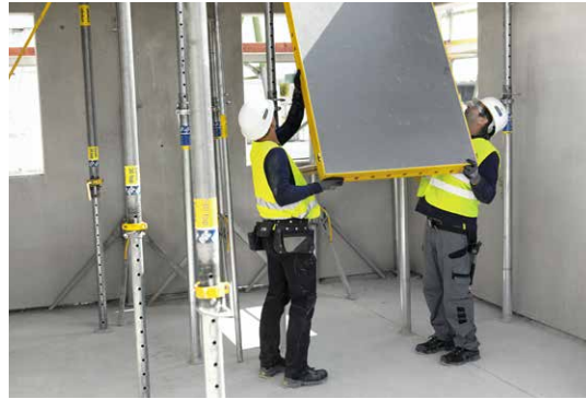
The DokaXdek panel floor formwork is a lightweight and flexible two-person element system.
