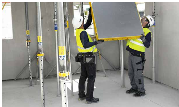
The DokaXdek panel floor formwork can be safely assembled from the ground.
