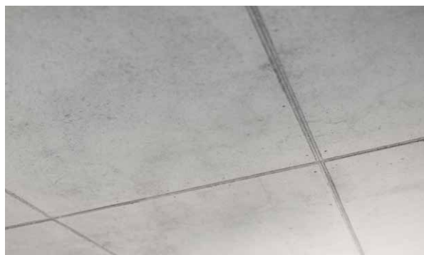
Good concrete result
