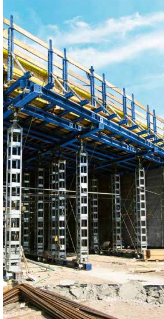
The SL-1 struts high load capacity greatly reduces the amount of shoring equipment needed, which also permits wide drive-through access openings.
