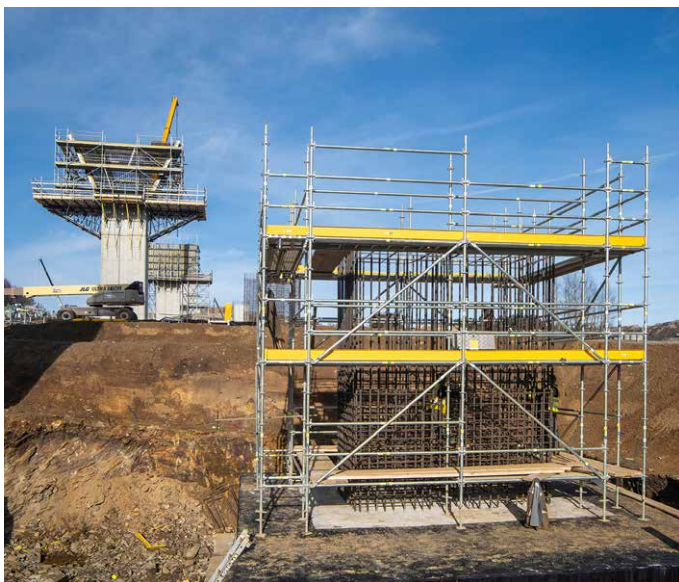
Ringlock rebar scaffold provides safe working platforms for steel fixers on Vystavda Estakada's bridge piers, Czech Republic.
