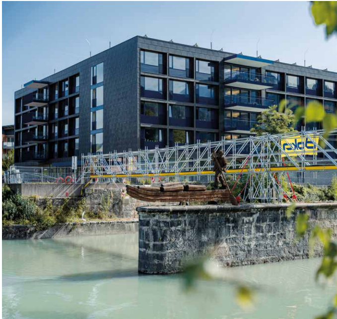
Ringlock as temporary cable bridge to cross the river in Hallein, Austria.
