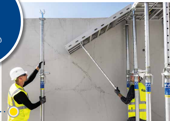
DokaXlight being tilted up
