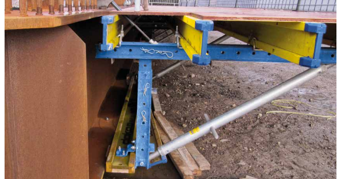
This versatile cantilever arm formwork is attached to the bridge superstructure by means of re-useable diagonal anchors.
