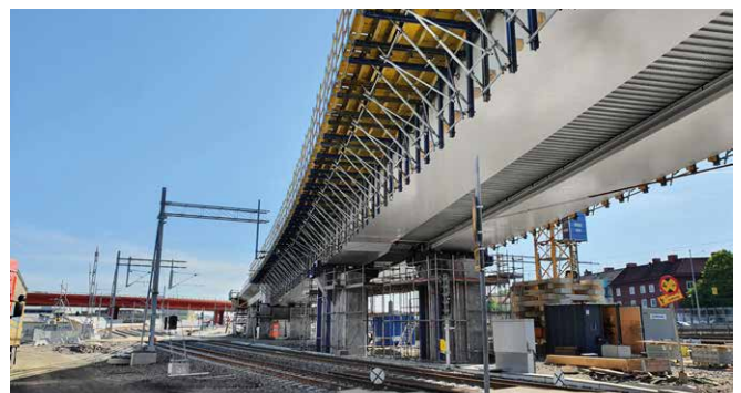
Flexibly adaptable – Optimized load distribution onto the steel structure during concreting.
