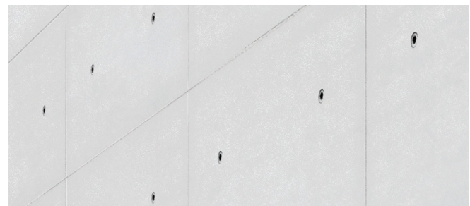
Appealing concrete surface
