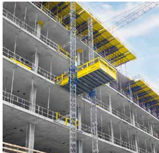
Fast construction workflows without the crane: with the Table Lifting System TLS, tableforms are brought up to the next floor at the push of a button.
