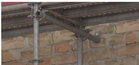
Figure 7.2: Example of tie member
