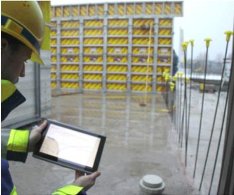
The **sensors** placed on the structure member continuously measure the heat development of the concrete, which is mainly influenced by the hydration heat of the cement and by ambient temperatures. The more intense the heat development, the faster the strength development of the concrete.
