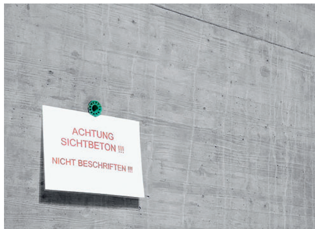
Protective warning sign for fair-faced concrete wall
