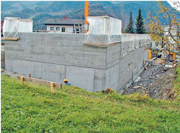
Protecting the starter bars (rust)
