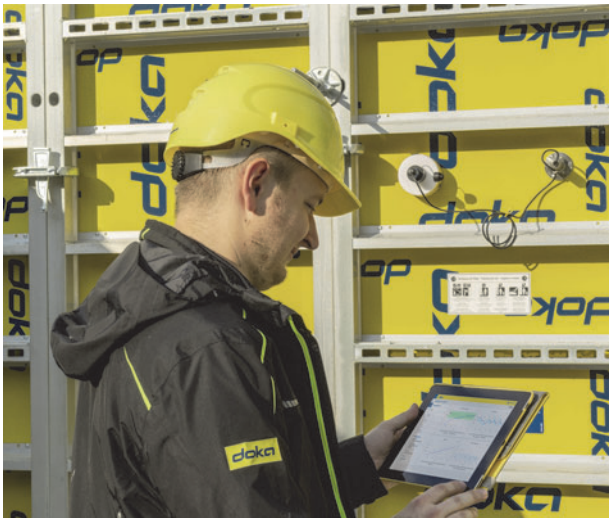
Use of the cable sensor
