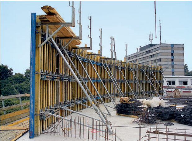
Screw-fixing of formwork sheeting at the edges (butt-jointing area) of the panels
