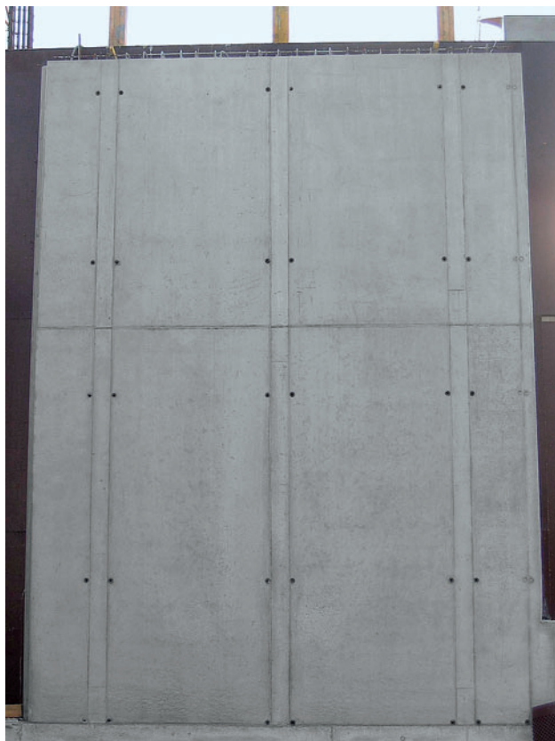
Same formwork sheeting (framed formwork and formwork sheet over fitting timber)
