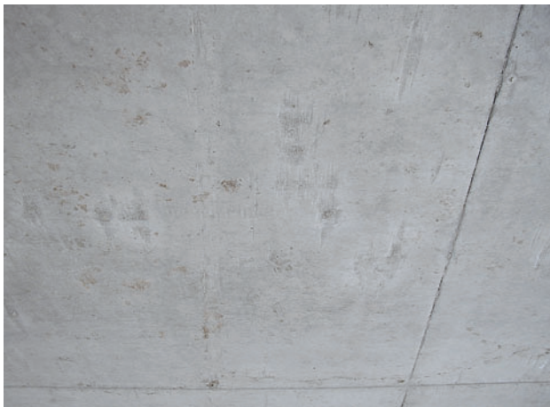
Slab showing vibrator damage
