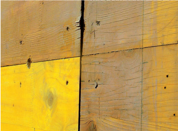
Example: Mismatch at the joint between adjacent panels
