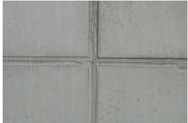
Frame imprint (width = 18 mm, depth = 1.5 mm)
