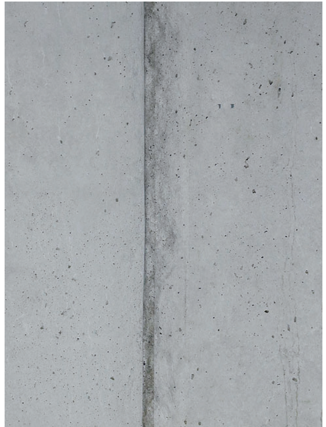
Construction joint made with sealing tape
