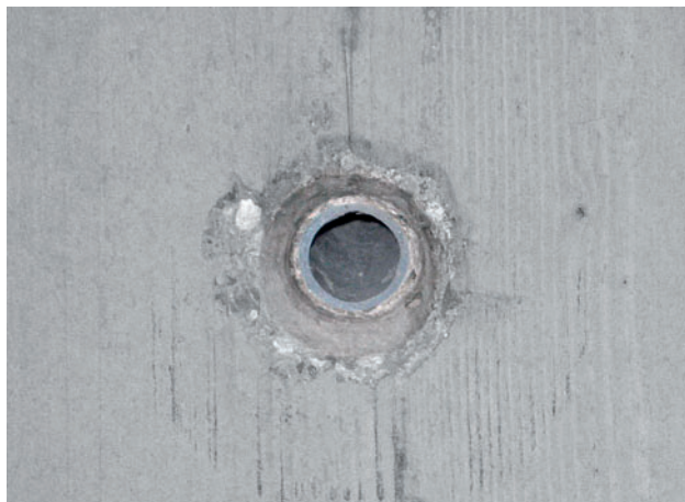
Edge-flaking around form-tie point
