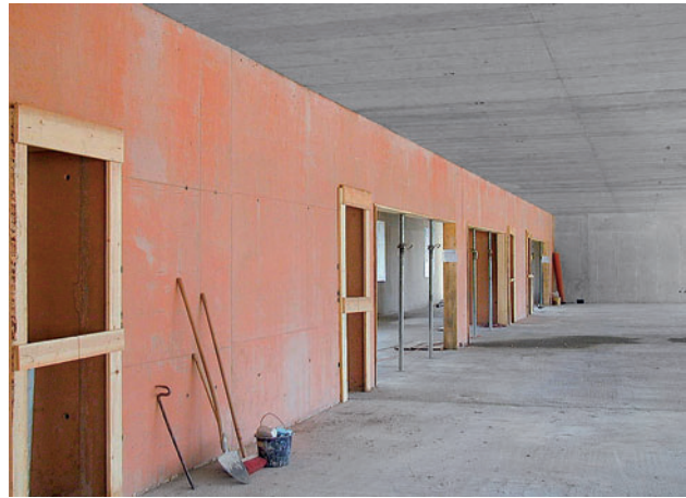
Edges protected, but lack of seal at the slab formwork
