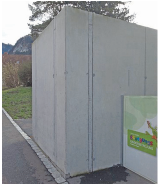
Frame imprint (width = 18 mm, depth = 1.5 mm)
