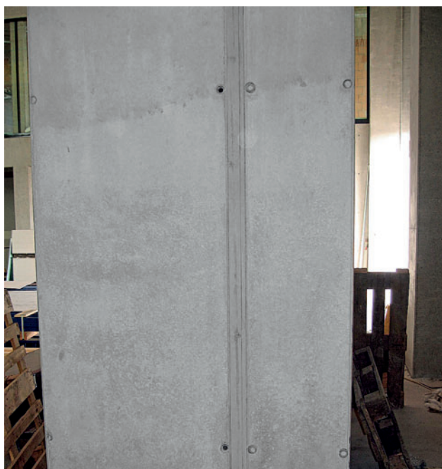
Different facing (framed formwork and fitting timber)
