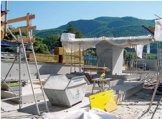
Protecting the starter bars (rust)
