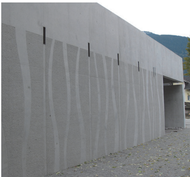
Treatment with concrete retardant followed by washing out of the treated areas
