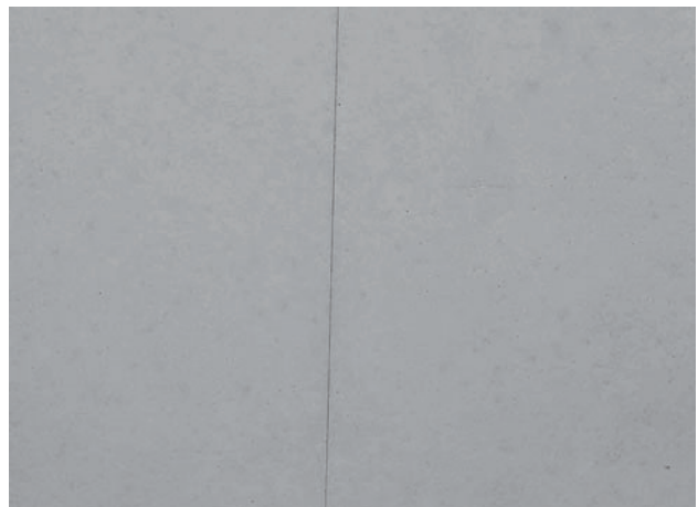
Appearance of concrete at joint (sealed) between sheets
