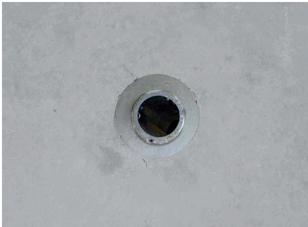
Sealed form-tie point with no bleeding and no edge-flaking
