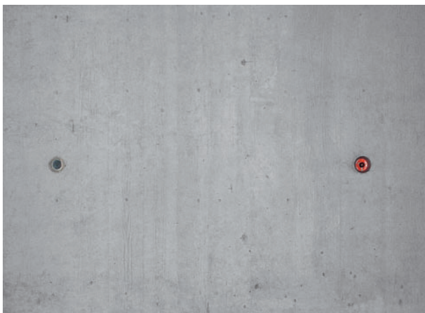
Uniform hole pattern (left: form-tie point - right: suspension point)
