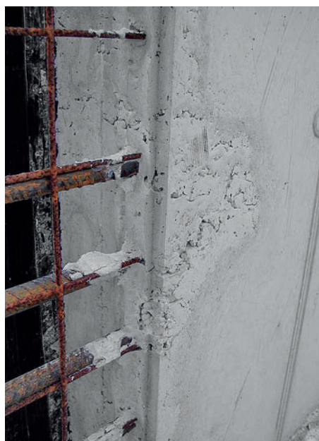
Result when stop-end formwork is not sealed
