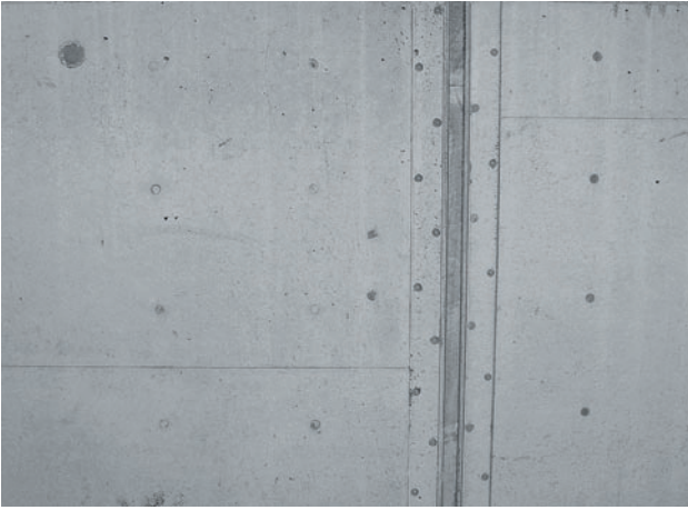
Screw-fixing of formwork sheeting at the edges (butt-jointing area) of the panels
