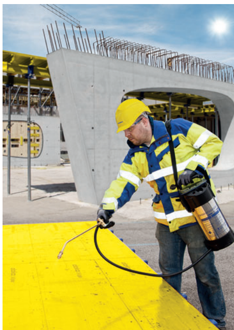
Spraying a formwork panel
