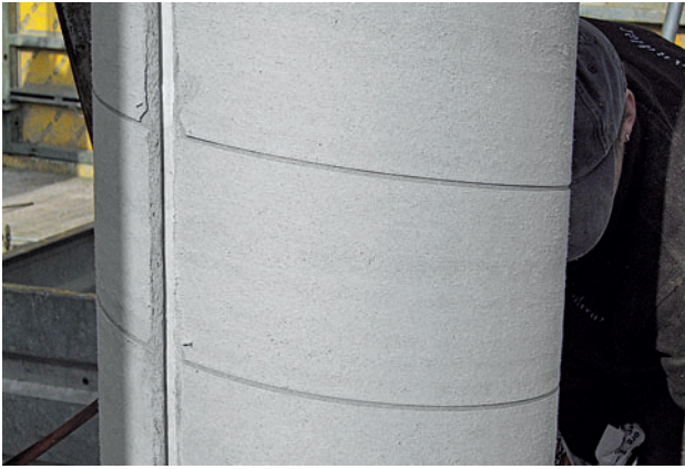
Concrete finish from standard version
