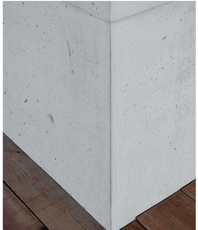
Corner cast without triangular ledge
