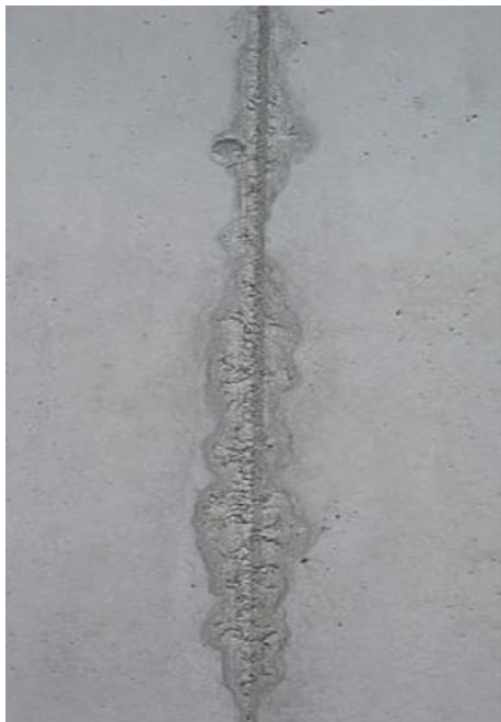
Seepage of cement slurry
