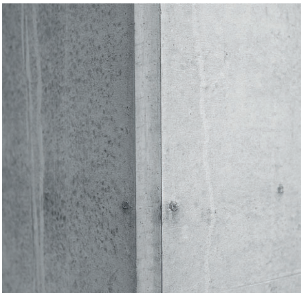
Corner cast with triangular ledge
