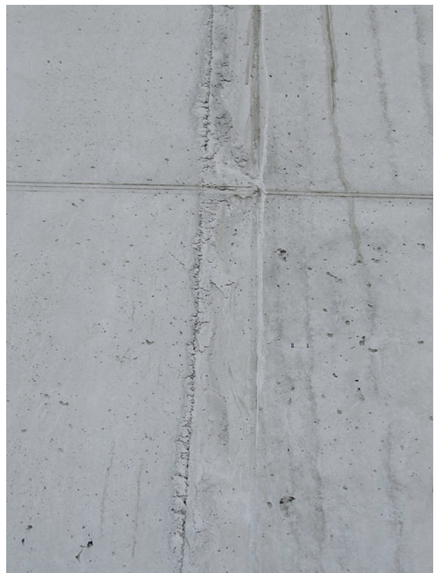
Construction joint made without sealing tape
