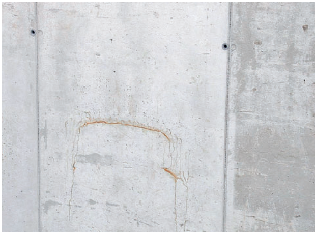
Soiling caused by condensation
