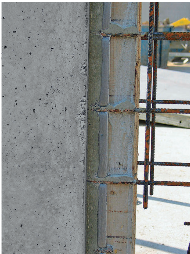
Stop-end formwork with sealing string
