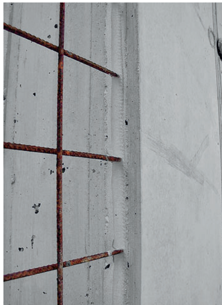
Result when stop-end formwork is sealed
