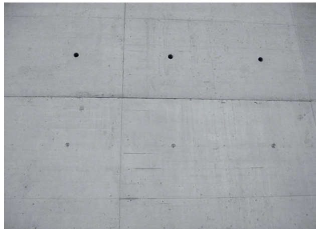
Horizontal construction joint cast with sealing tape
