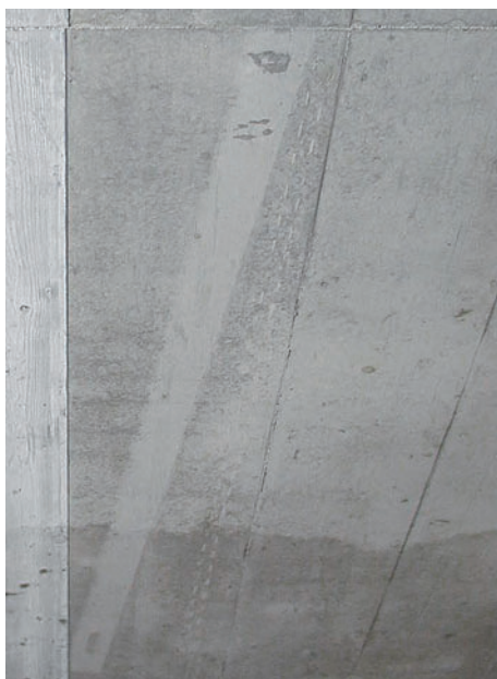
Concrete discolouration caused by an aluminium levelling rule being left on the formwork sheeting
