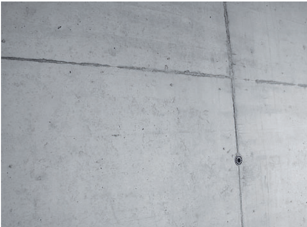
Appearance of the concrete due to mismatch at the joint between adjacent panels
