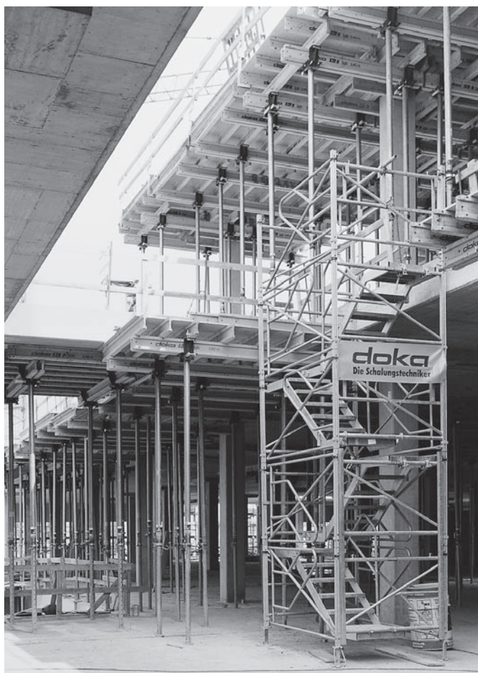
Obra: ARGE Westmünster Center, Bocholt
