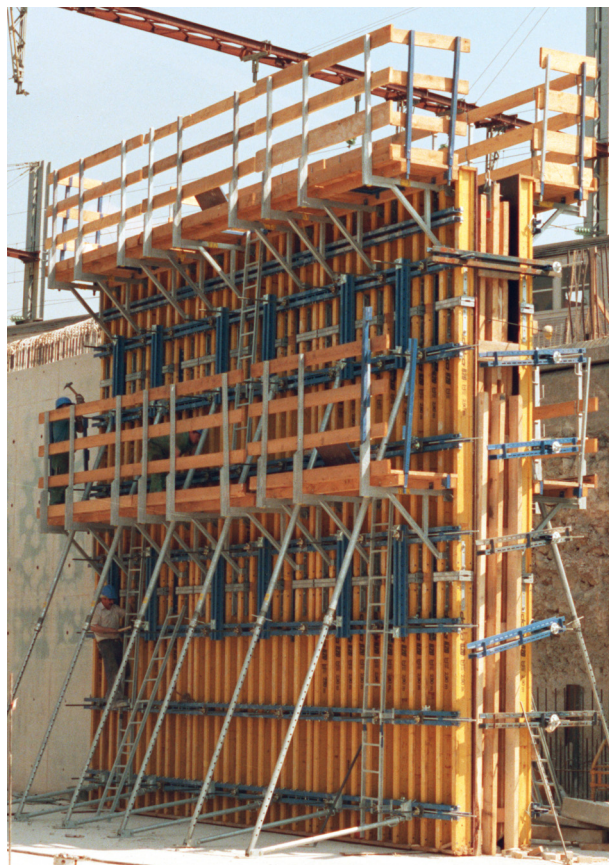
Obra: TVG Nord Bridge No. 4, Paris
