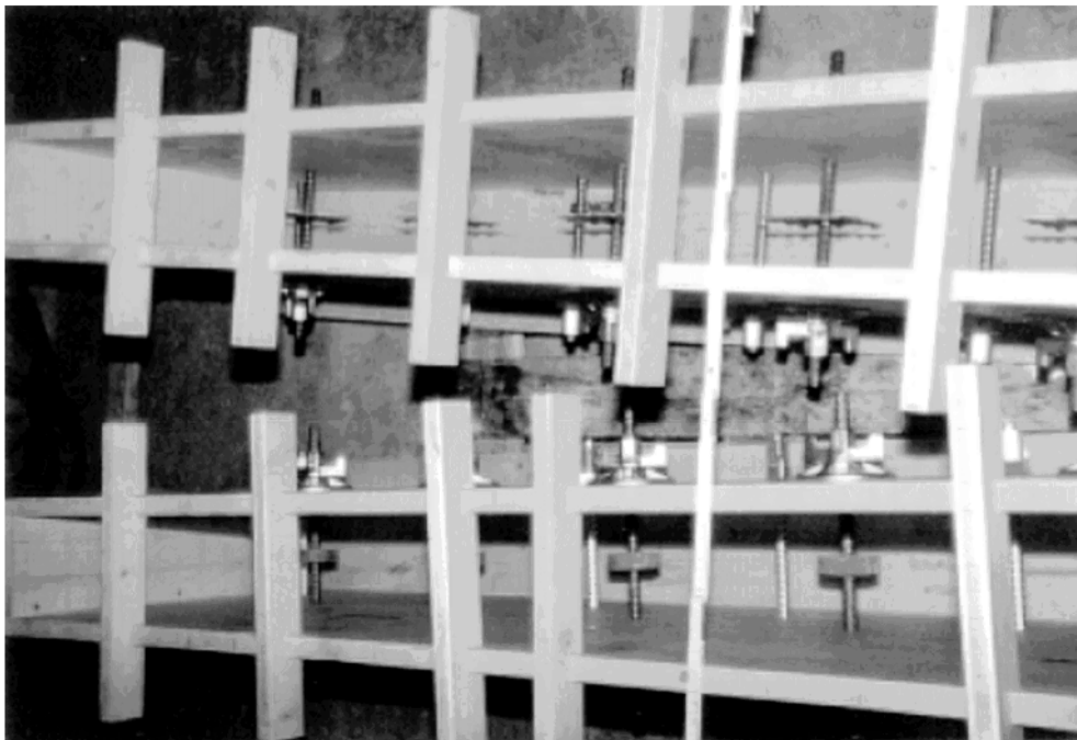
Fig. 3: View into the formwork showing the different types of form-tie (at left: Water stop 15.0 and tie-rods, galvanised; at right: Water stop G 15.0 and tie-rods, non-treated)
