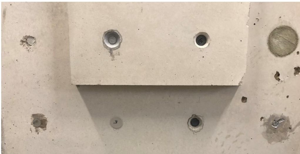
Fig. 12: Detail of form-tie points 1 to 8 of side 2
